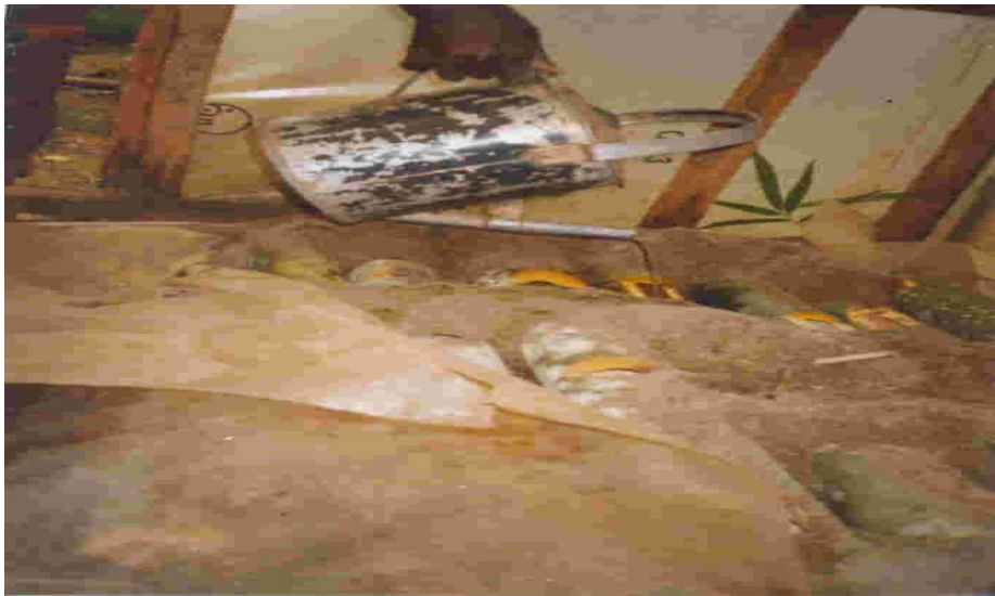
Plate 6: Filling holes with mixture of water and fungicide
