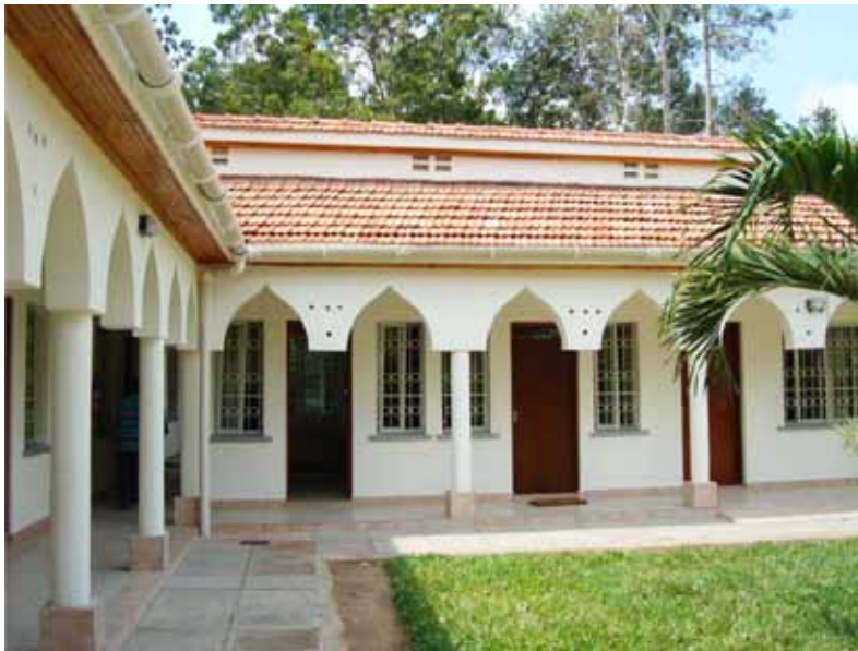
Research facility for the Coastal Eco-region Forestry Research Programme - Gede
